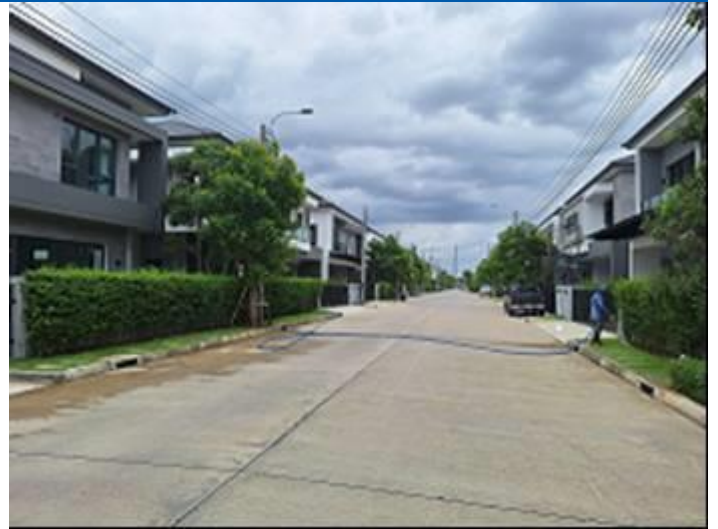
Figure 6: Complete SDH units on the project's main road available for transfer
